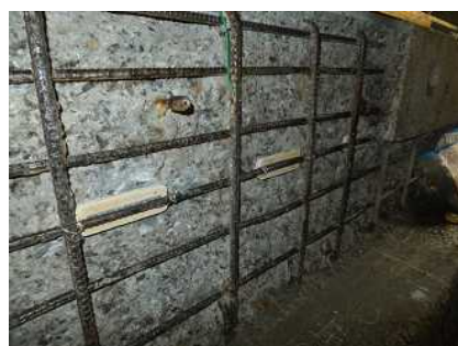
写真-5.5 犠牲陽極設置状況
