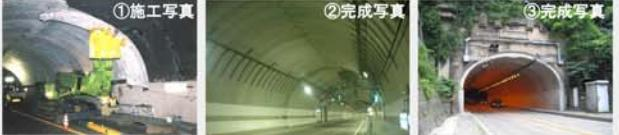
PCL 工法® -Precast Concrete tunnel Linings
