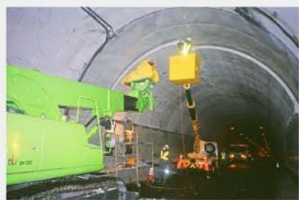
PCL 工法® -Precast Concrete tunnel Lining
