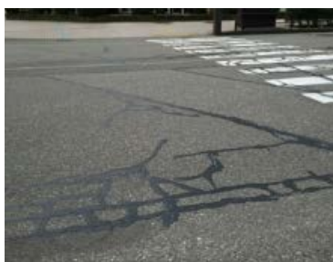
Figure 4: Crack sealing
