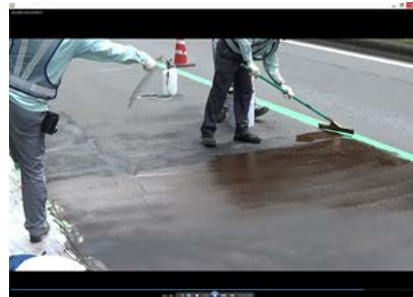
Figure 5: Thin layer surfacetreatment
