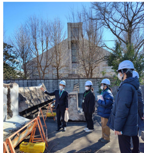
Photograph 2: Deteriorated concrete girders
