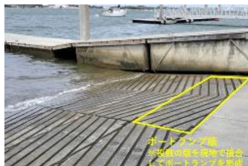
Photograph 6: Boat ramp slabs at a port facility.
