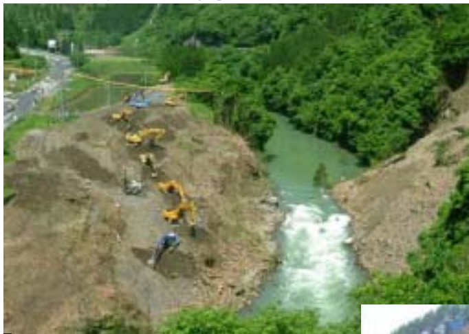
Picture 4 River widening on the opposite bank of the river
