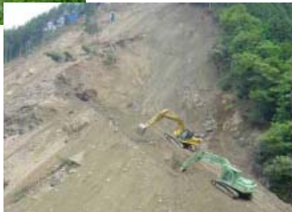
Picture 5 Emergency earth removal using remote-controlled machinery
