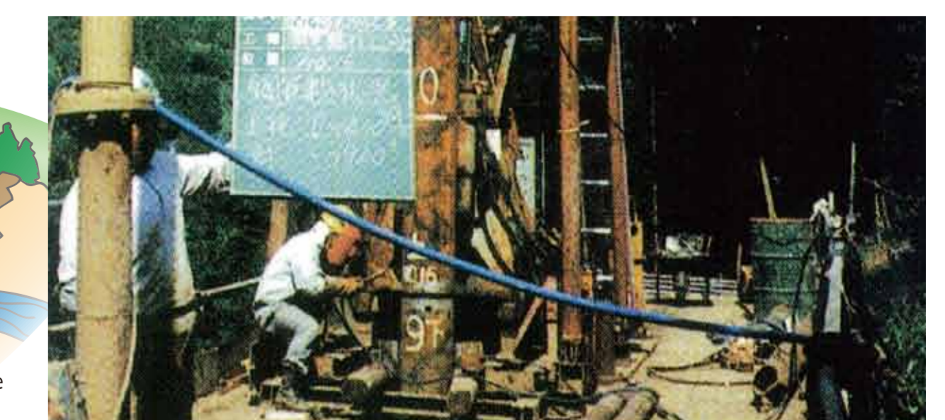
▲杭工 Piling works
