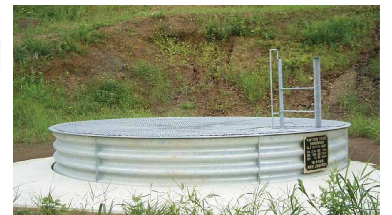
▲集水井工 Water catchment well works
